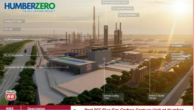
Post FCC Flue Gas Carbon Capture Unit at Humber H00 Plot Enabling Refinery. H01 Flue Gas Supply Design Capacity 0.5 MMTPA to recover & purify 95% H02 Pre-Treatment Absorption & Regeneration
